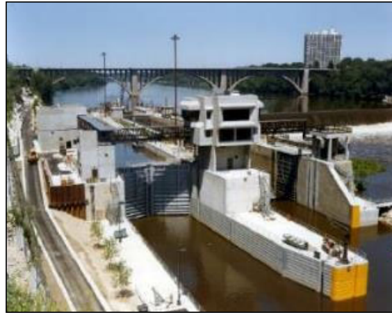
Lock and Dam No. 1 (L/D 1)
